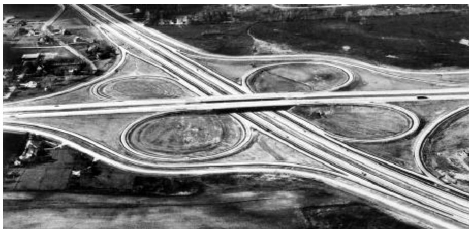
Exhibit 10-26. Four-Leg Interchange, Full Cloverleaf With Collector-Distributor Roads
