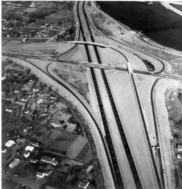
Exhibit 10-39. Four-Leg Interchange, Diamond With a Semidirect Connection
