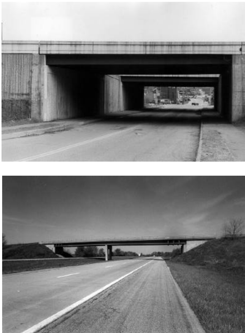
Exhibit 10-3. Typical Grade Separation Structures With Closed Abutments
