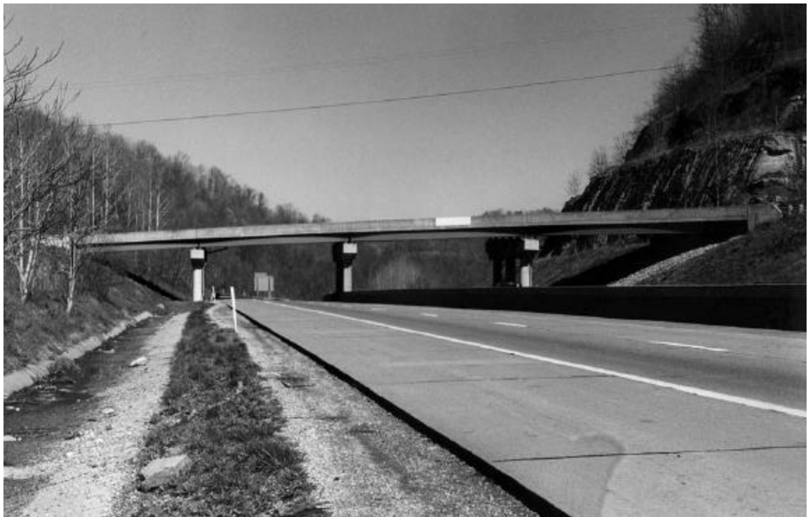
Exhibit 10-4. Typical Grade Separation Structure With Open-End Span
