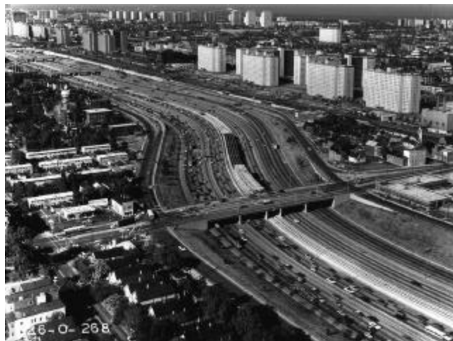
Exhibit 8-25. Dual-Divided Freeway With a 4-3-3-4 Roadway Arrangement
